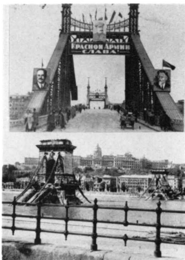
Above: Communist-held bridge crossing the Danube in Prague. Below: The Budapest Chain Bridge over the Danube, in ruins in 1948.
